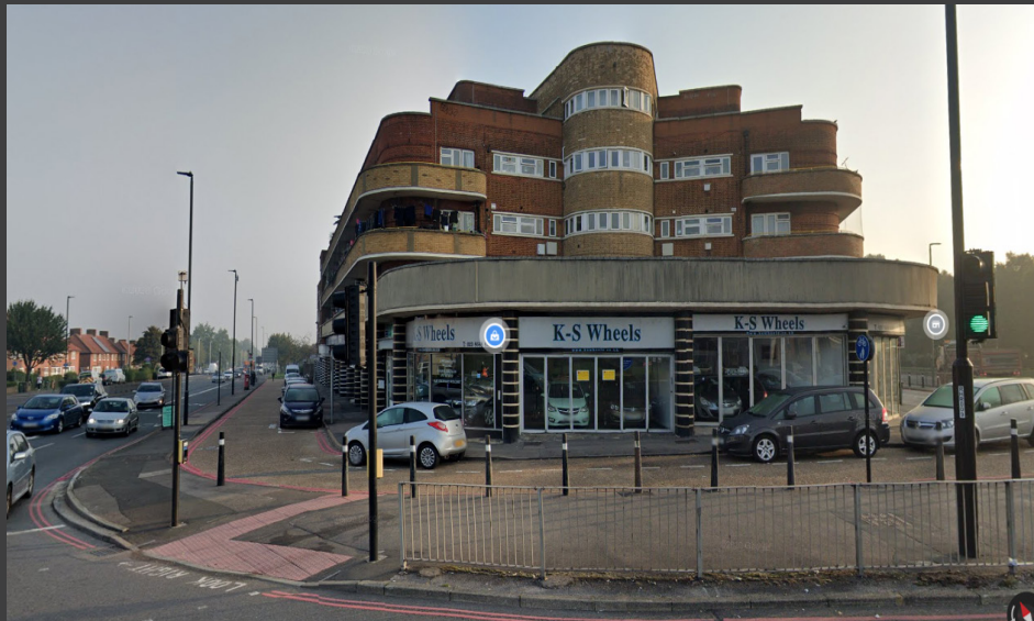
1. Rosehill Court viewed from the north of Rose Hill roundabout
