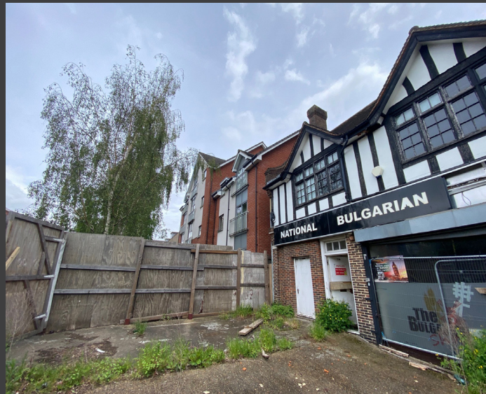
2. View of Renaissance Court from the site looking north
